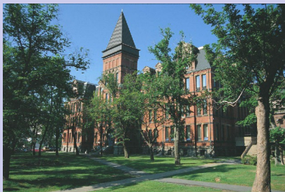
Forrest Building, Dalhousie University
